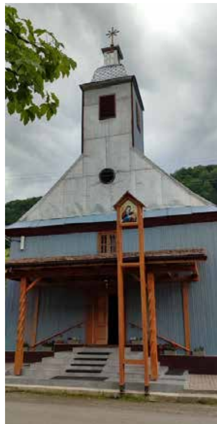
Photo 11. The modern appearance of the church, changed, covered with metal instead of shingles, the original appearance has not been saved [2; 4]
